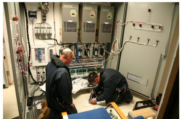
Figure 2 - The motor control cabinet being wired and tested in the old LAMA room.
