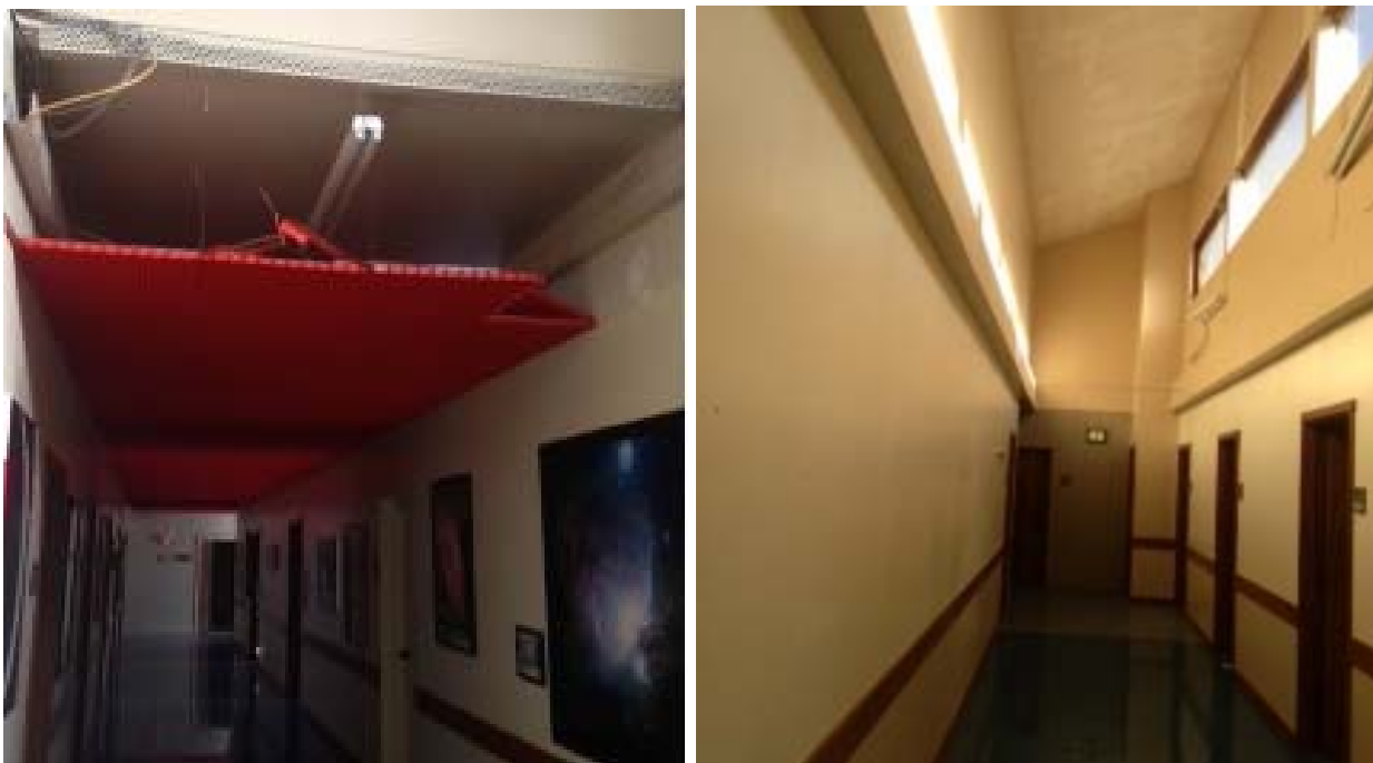
Figure 21 – The interior of the Waimea office is getting a facelift by removing all of the original orange metal ceiling material (left), letting in much more natural lighting and taking advantage of the high ceilings originally designed into the building (right).
