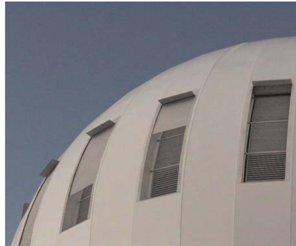
Figure 12 - A rendering showing how four of the twelve vent units and their associated ice deflectors, rollup weather doors and internal louver vanes will look after installed in 2013.
