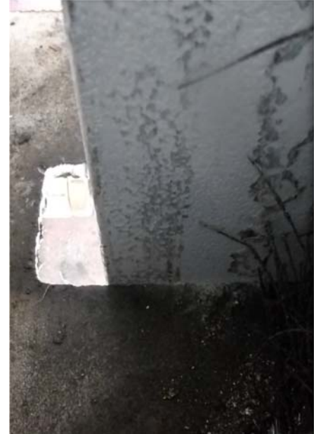
Figure 9 – This close up view of an "ice wiper", deep within the shutter assembly, was found to be in contact with shutter rail, contributing the shutter jamming for several weeks in early 2013.
