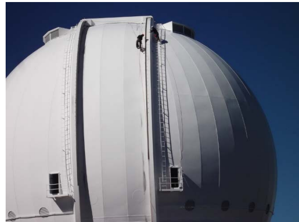
Figure 10 – Staff from Climb Aloha are seen repelling down the CFHT dome as part of the on-going repairs to the dome shutter drive system.
