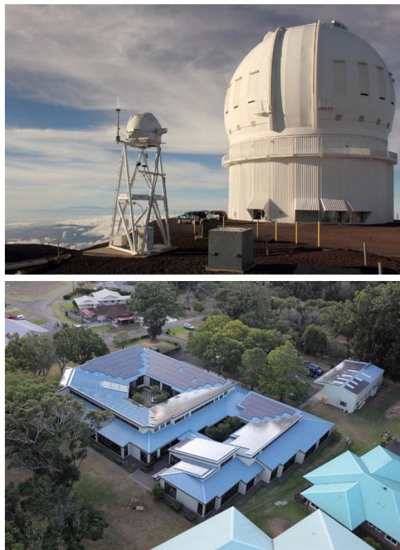
Figure 1 – Top: The new dome vents, soon after installation. Each vent is independently configurable and the curved inset design beautifully matches the contours of the dome. Bottom: A photo taken from a kite-mounted DLSR showing the ~600 solar PV panels on the roof of the headquarters office and shop in Waimea. Images courtesy Tom Benedict
