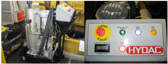
Figure 14 – The new HYDAC water removal system for the summit hydraulic supply is shown.
