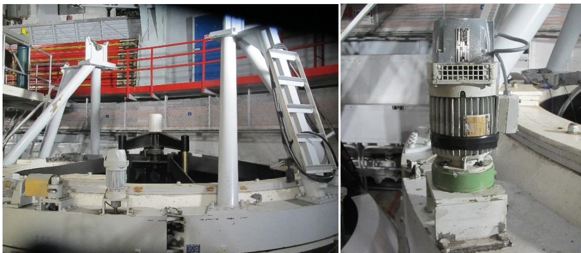
Figure 20 - (Left) Handling ring gate segment shown. (Right) Gate segment motor/brake/gearbox repaired.
