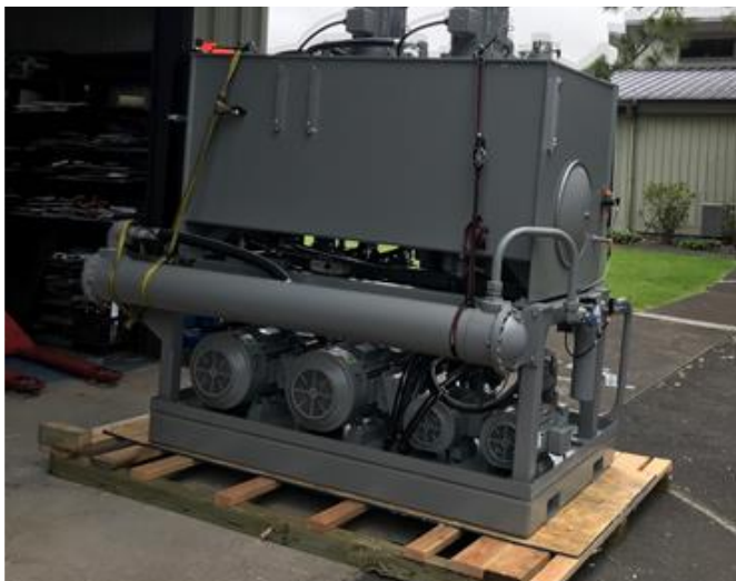
Figure 11 - The completed new hydraulic power system in Waimea.
