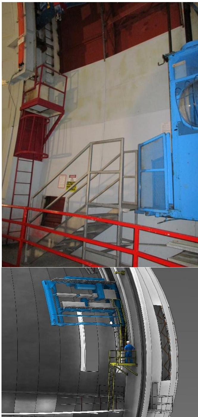
Figure 14 - (top) Existing bridge crane access and (bottom) SolidWorks model of new crane access.
