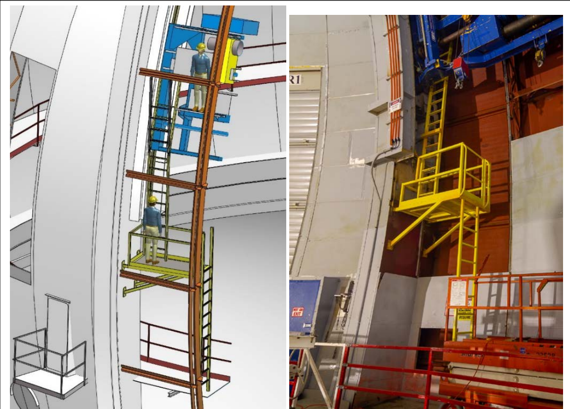
Bridge crane access platform: design (Left) installation (Right).
